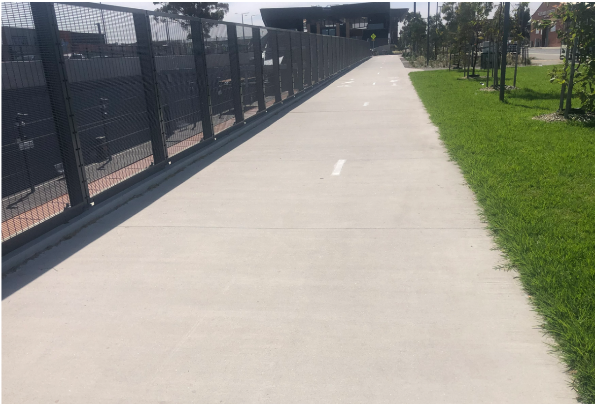
Photo 7: Shared Path alongside the Craigieburn Line Rail cutting
