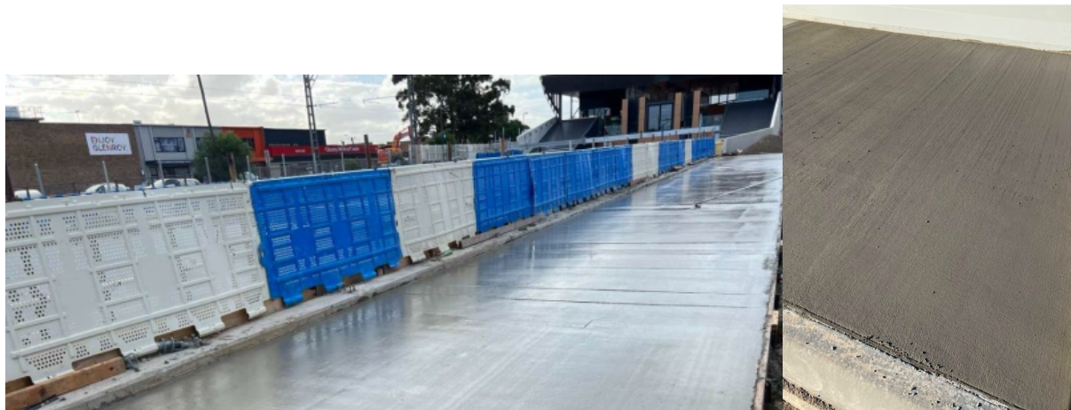
Photo 4: Concrete after finishing; Photo 5: Broom finish applied during construction
